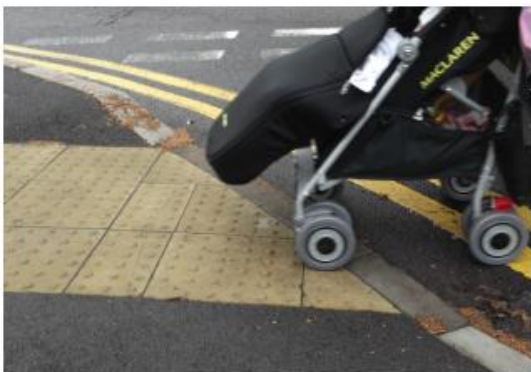
Dropped kerb with tactile paving
